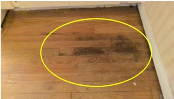
Stained wood flooring
