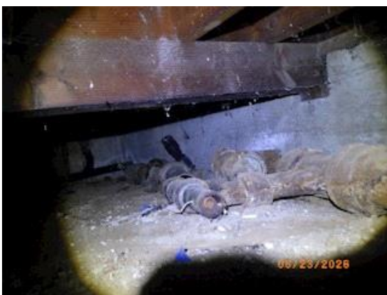
Dismantled old plumbing system debris
