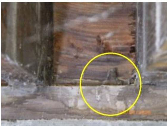
Anchor bolts confirmed
