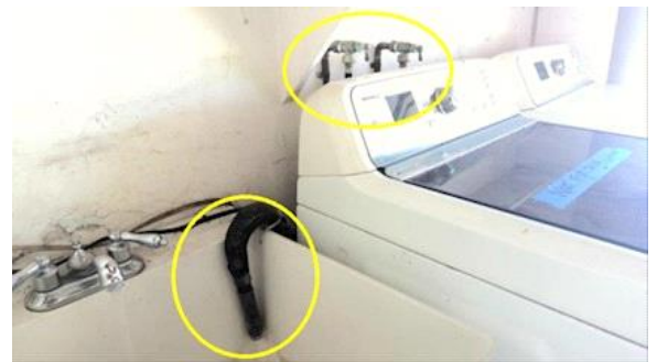
Laundry hookups & laundry tub drainage intact
