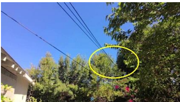
Overhead service entwined with tree limbs
