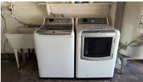
Confined Laundry area / Unconfirmed existing machines
