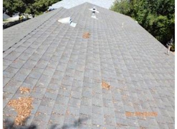
Roof top view #3
