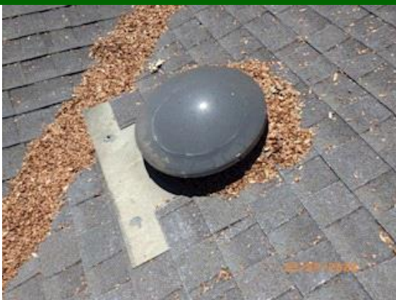
Overview of intact roof top assembly
