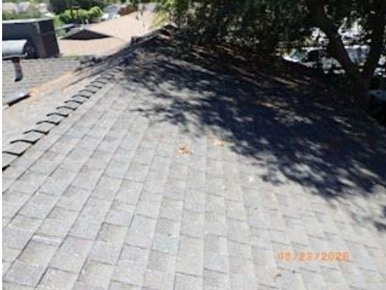
Roof top view #2
