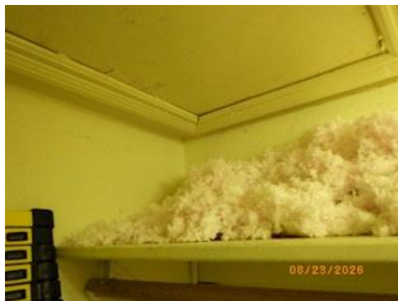
Obstructions @ attic entrance
