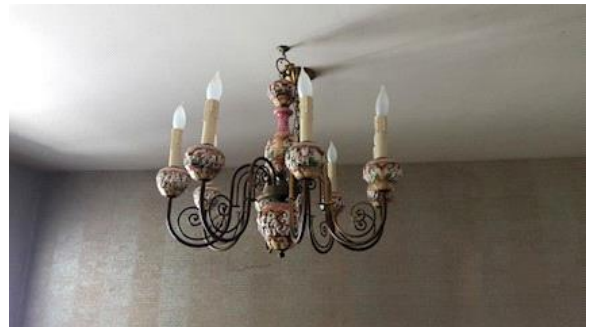
Unconfirmed / inoperable light fixture
