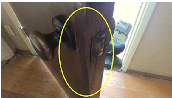
Cracked front door edge
