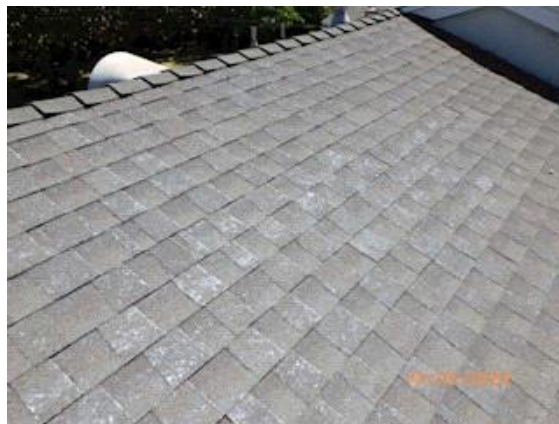
Roof top view #1
