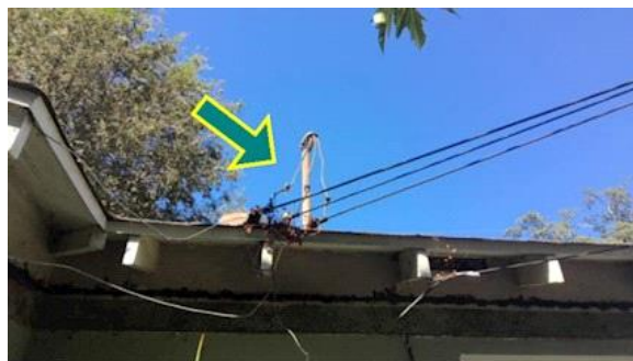
Observed overhead main service intact
