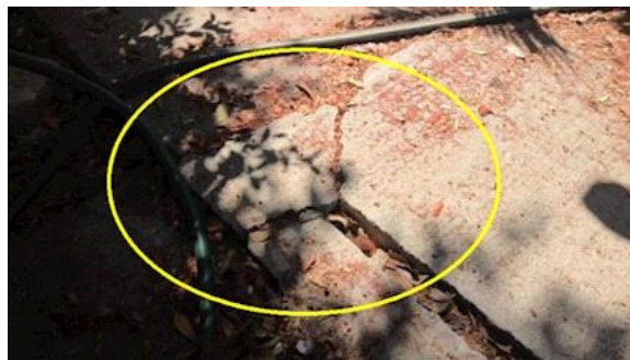
Cracked concrete
